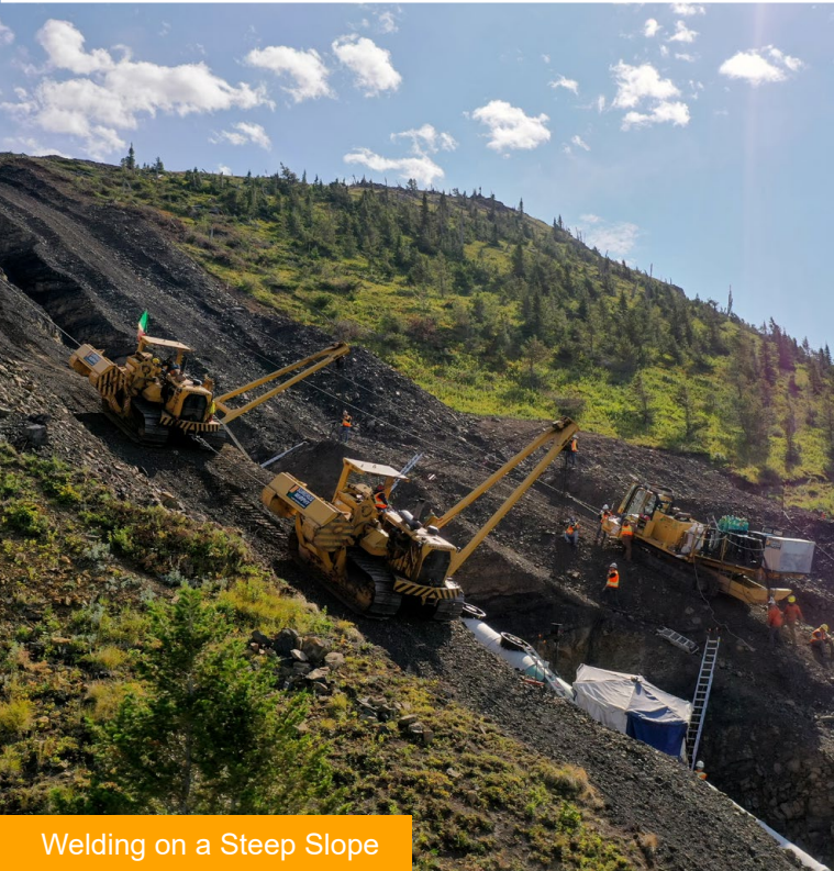
Automated Tie-In Welding on Above-Ground Pipeline Loop
