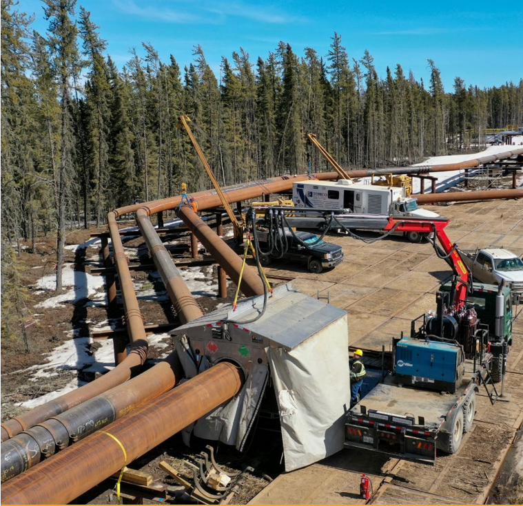
Automated Tie-In Welding on Above-Ground Pipeline Loop
